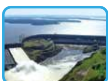
Hydro-Electric Power Generation
